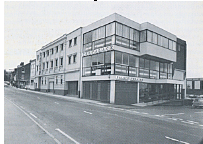
Palace Theatre (as renovated by Development Corporation in 1971)
